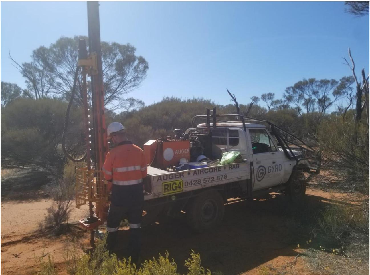
*Figure 1: Auger sampling underway at Yarbu Gold Project*
